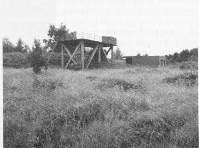
Bloodhound radar platform and building
